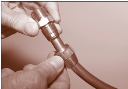
FIGURE 28: Flare Fitting/Flared Joint During Assembly
