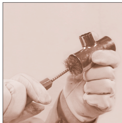
FIGURE 17: Cleaning: Fitting Brush
